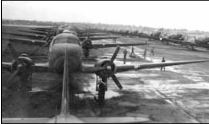
Left: C-47 aircraft are parked on each side of an extended runway in preparation for a glider-tow. The gliders were towed to the center of the runway by a tug and the tow aircraft waved into place at the end of the towrope. Care was taken by the towing aircraft to gain speed without breaking the towline. The glider and tow plane maintained contact through an intercom line.
