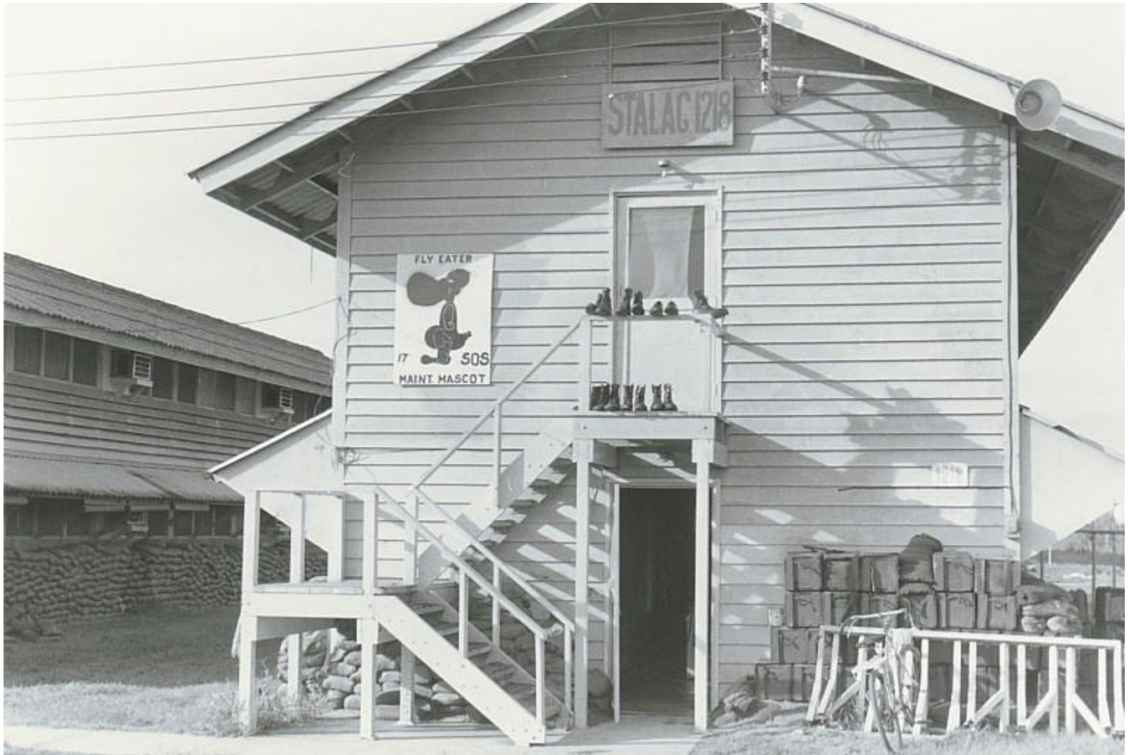
MAINTENANCE BARRACKS – TAN SON NHUTMAI
