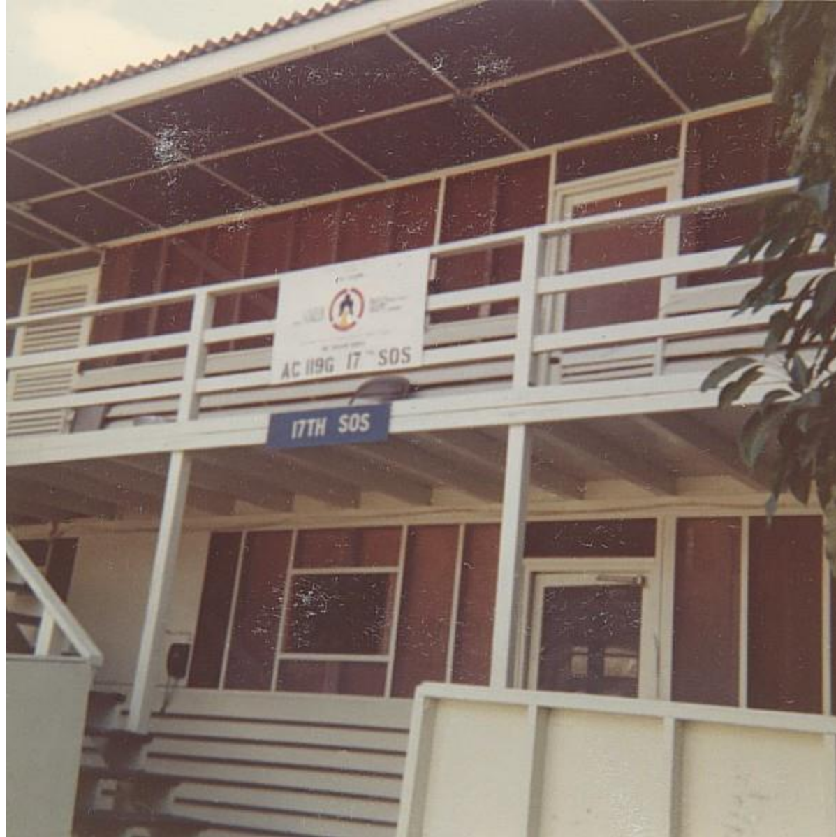
MAINTENANCE BARRACKS – PHU CATM
